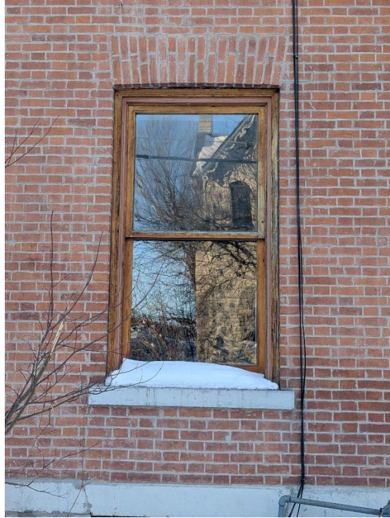
Top Image: Existing main floor window on the southeast (front) façade..
