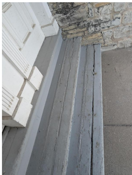
Existing conditions of carriageway entrance. Concrete landing and wooden steps.
