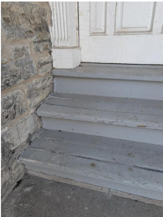
Existing conditions of carriageway entrance. Concrete landing and wooden steps.
