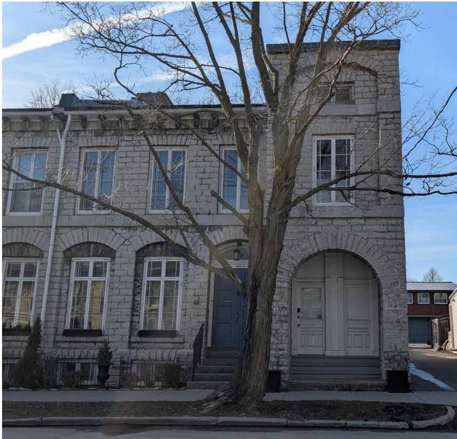
Bottom Left Image: Southeast (front) façade of 226 King Street East.
