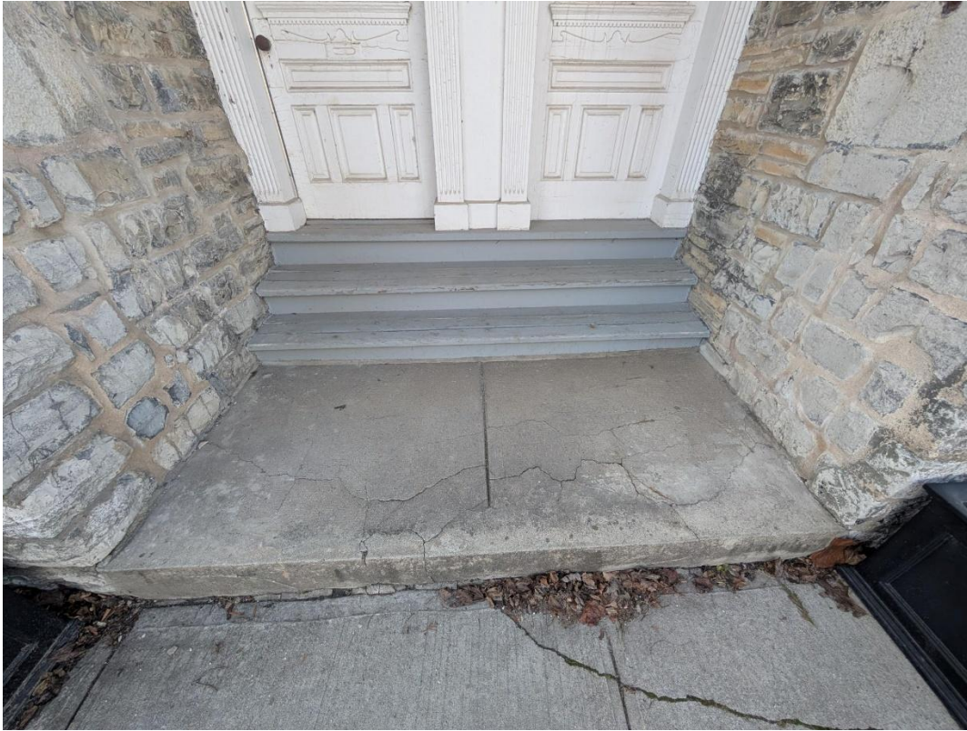
Existing conditions of carriageway entrance. Concrete landing and wooden steps.
