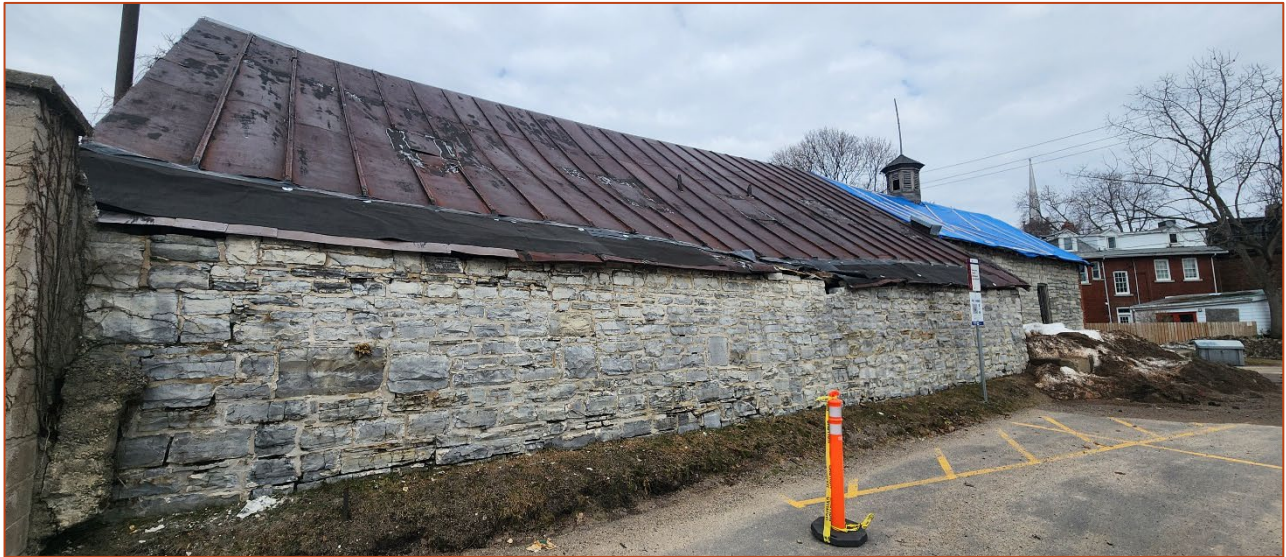
Photo 5. View of the south elevation of the addition
