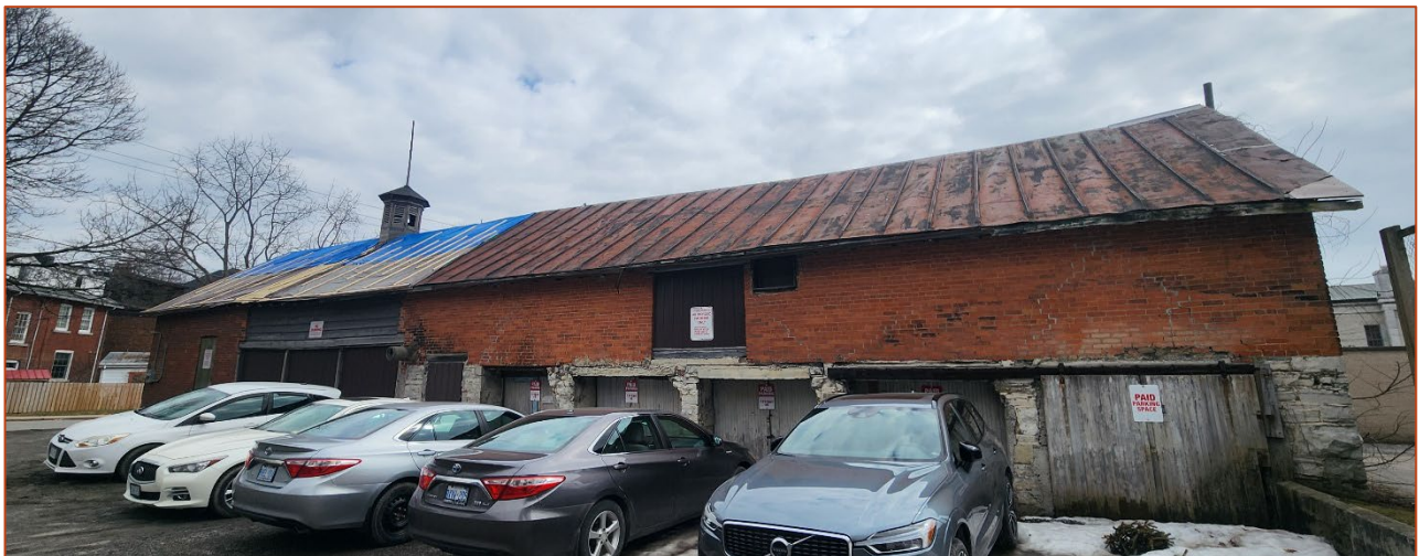
Photo 4. View of the north elevation
