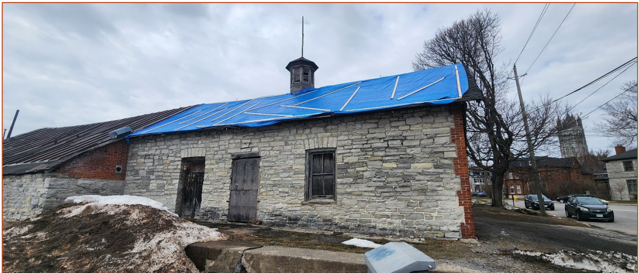
Photo 2. View of the south elevation
