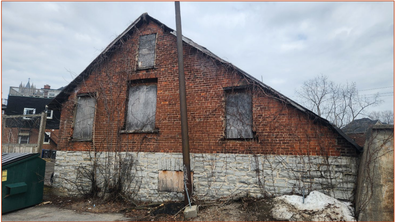
Photo 3. View of the west elevation of the rear addition
